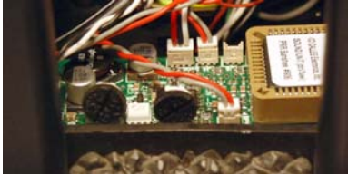
Looking into the front access panel of the tender at the sound unit.
